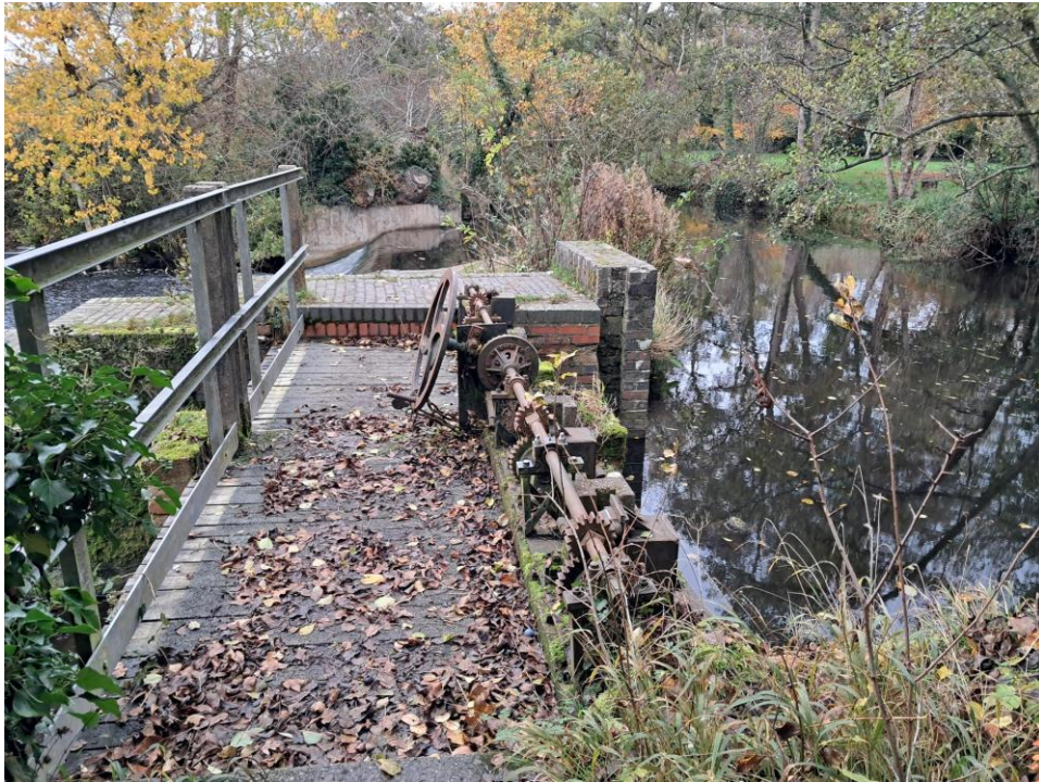
Image 5. Site photograph of Island Meadow Caravan Park sluice gate control. Note: impounded river above the weir continues to flow south into the mill leat in the right of this image.
